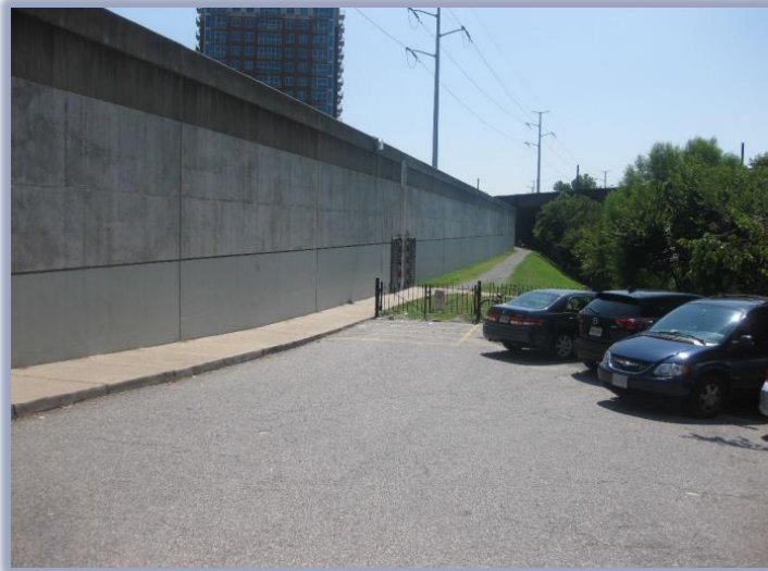
Example of T-Wall provide by Army Corps. Height of this wall not known.
